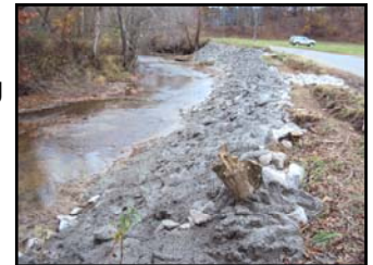
Streambank Revetment Project – Blue Rock
